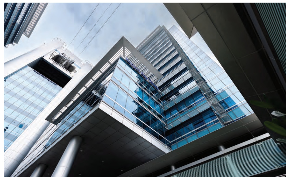
Keppel Land is seizing opportunities in sustainable urban renewal. (In picture: Keppel Bay Tower, Singapore's first BCA Green Mark Platinum (Zero Energy) commercial building.)
