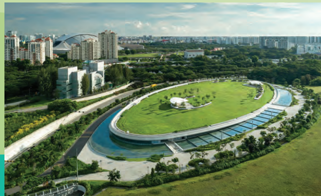
Keppel Marina East Desalination Plant, Singapore
