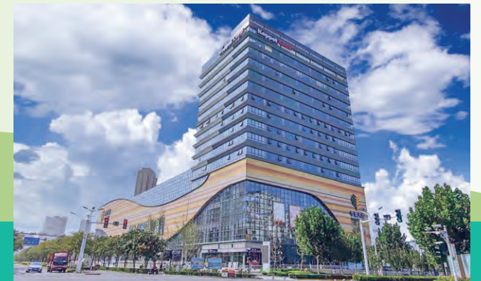
Seasons City retail mall in Tianjin, China
