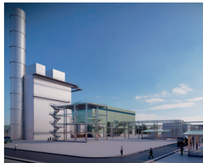
The global transition away from fossil fuels and towards zero- and low-emission technologies bodes well for many of the solutions that Keppel provides, including renewables and the development of the Keppel Sakra Cogen Plant, Singapore's first hydrogen-ready and most advanced power plant (in picture).
