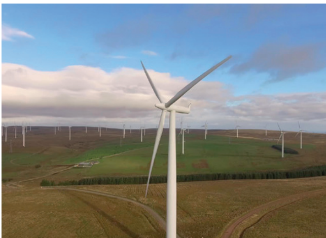
To tap the growing demand for renewable energy, Keppel, together with Keppel Infrastructure Trust (KIT), jointly acquired a 16.3% stake in Fäbodliden II, a 17 MW Swedish onshore wind farm. The acquisition follows an earlier joint investment made by Keppel and KIT alongside partners, for a 49% share of an initial portfolio of onshore wind energy assets (pictured) across Norway and Sweden sponsored by Fred. Olsen Renewables AS (FORAS).
