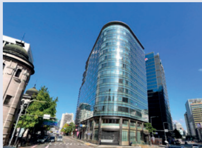
Keppel applies its Sustainable Urban Renewal (SUR) solutions to enhance the efficiency, sustainability performance and valuation of its real estate assets under management. (In picture: The Bank of Korea's Sogong Annex Facility in Seoul, which is undergoing SUR asset enhancements.)
