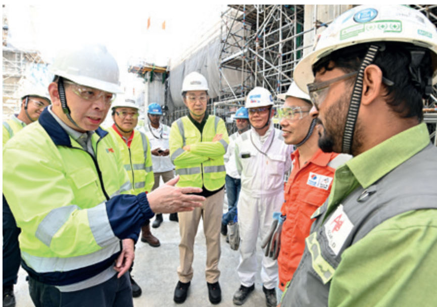
In 2023, the BSSC visited the Keppel South Central project site, as well as the construction site of the Singapore Integrated Waste Management Facility.
