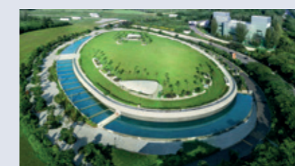
Keppel Marina East Desalination Plant Singapore's first large-scale, dual-mode desalination plant that treats both rainwater and seawater
