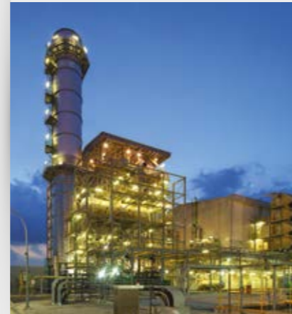
1.3 Combined-cycle gas turbine power plant
