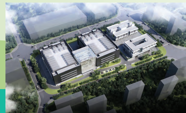
Data centre in Huizhou, China
