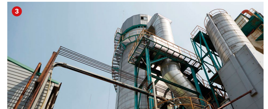
Expanding capabilities in environmental infrastructure.
