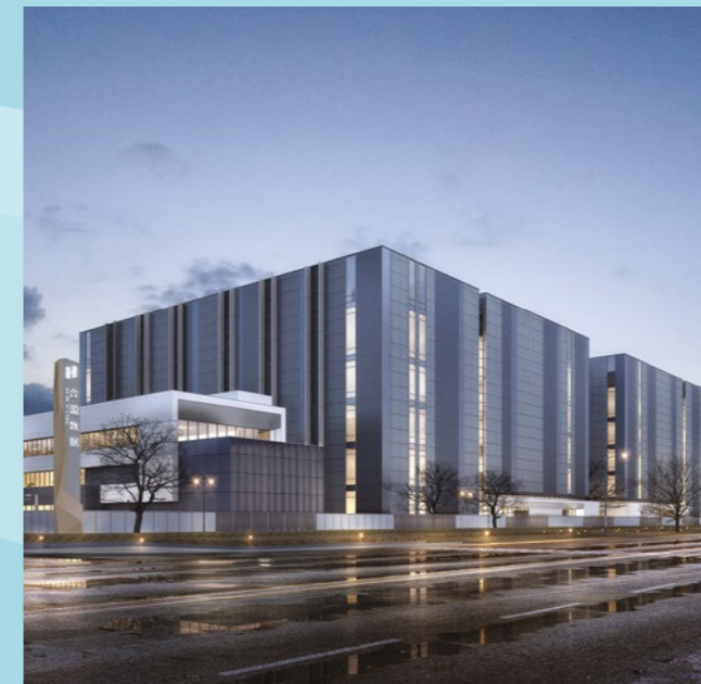
Data centre in Greater Beijing, China
