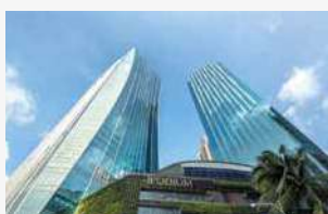
The Podium development is envisioned to serve the growing demand for prime office spaces in Manila, the Philippines.
