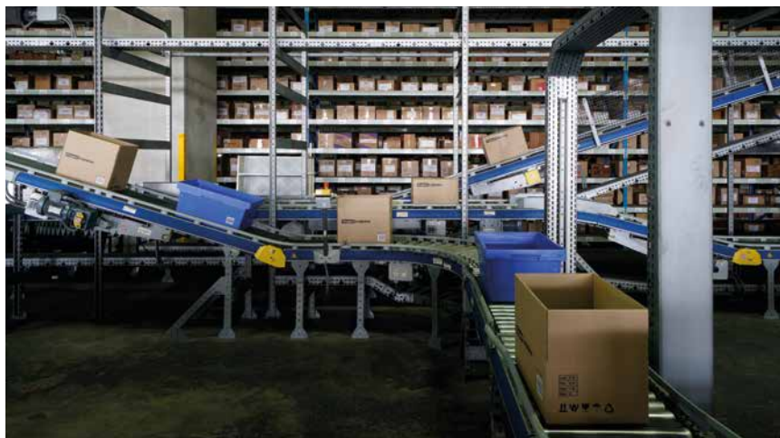
During the year, Keppel Logistics built new capabilities and expanded its omnichannel solution offerings to customers in SEA.
