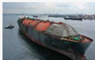
Keppel O&M received final notice to proceed for the conversion of the Gimi FLNG.
