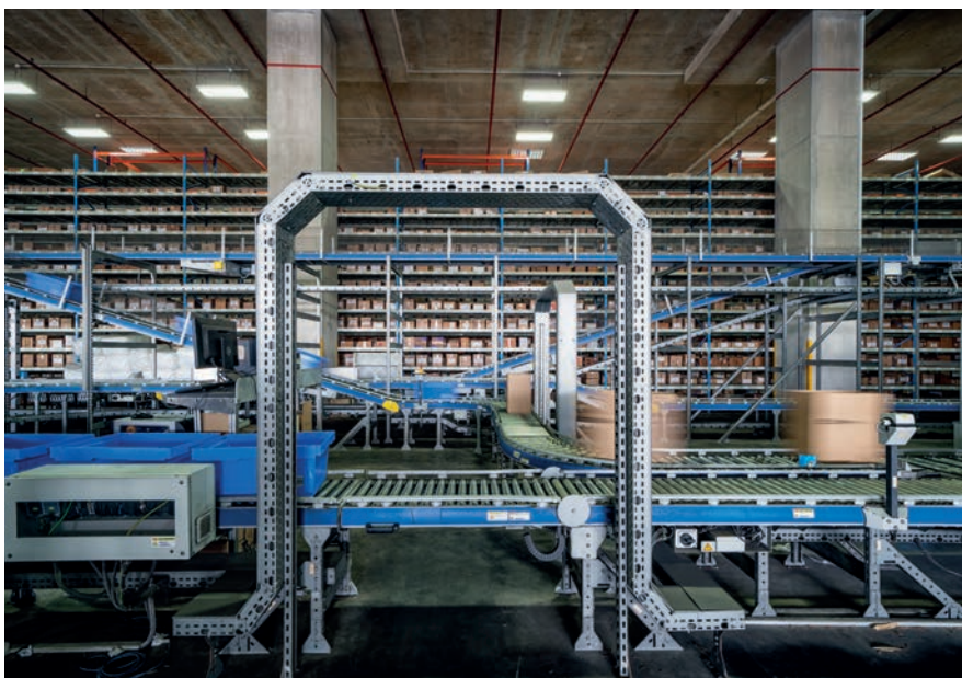
During the year, Keppel Logistics fully integrated its B2B and B2C operations at Tampines Logistics Hub in Singapore, and expanded its omnichannel solution offerings to customers in SEA.
