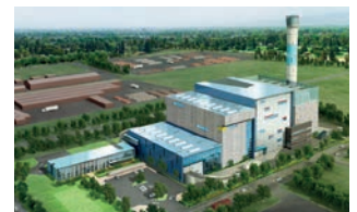
Australia's first WTE plant in Kwinana will use Keppel Seghers' proprietary technology and processes.
