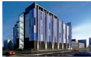
Intellicentre 3 East Data Centre is Keppel DC REIT's fourth data centre in Australia.
