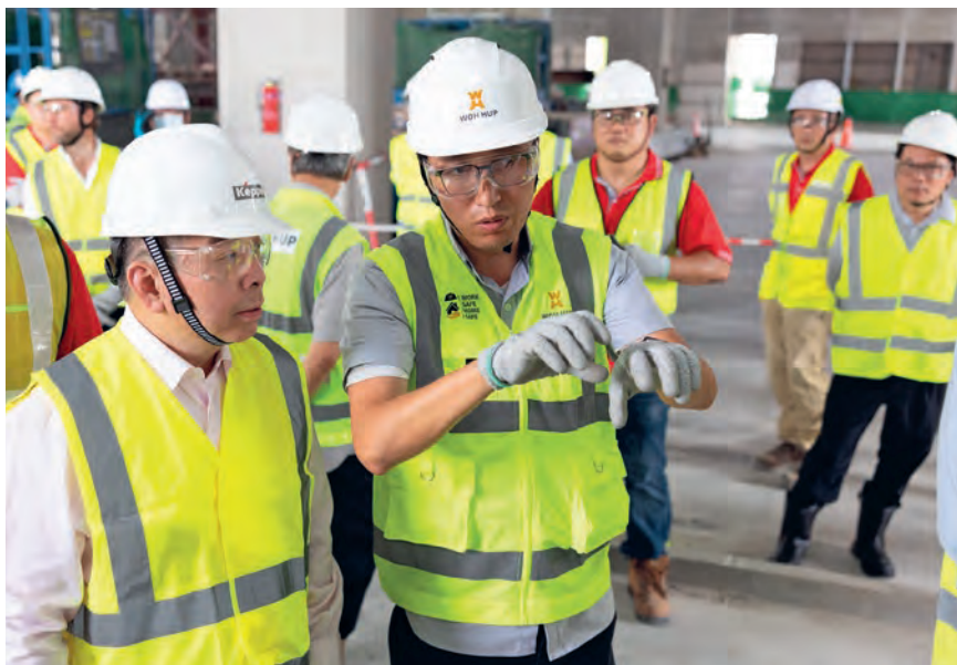
In 2024, the BSSC conducted visits to the construction sites of Keppel Data Centre Singapore 8 (in picture) at Genting Lane and Keppel South Central in Singapore, as well as the construction site of the Inno88 Tower in Seoul, South Korea.
