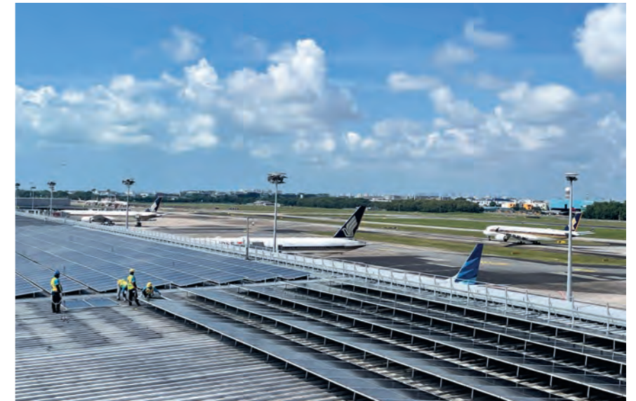
International efforts to decarbonise and combat climate change will drive demand for Keppel's Energy-as-a-Service solutions. (In picture: Singapore's largest single-site rooftop solar photovoltaic system at Changi Airport designed, built and being operated by Keppel over 25 years.)
