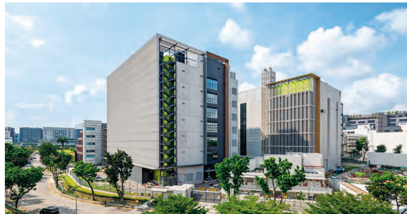
Connectivity will continue to be a growth sector, with digitalisation and Generative AI driving demand for subsea cables, energy-efficient data centres, such as the Keppel Data Centre Campus (in picture), and digital connectivity solutions.
