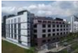
Keppel DC Singapore 1*
