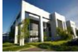
Keppel DC Dublin1*
