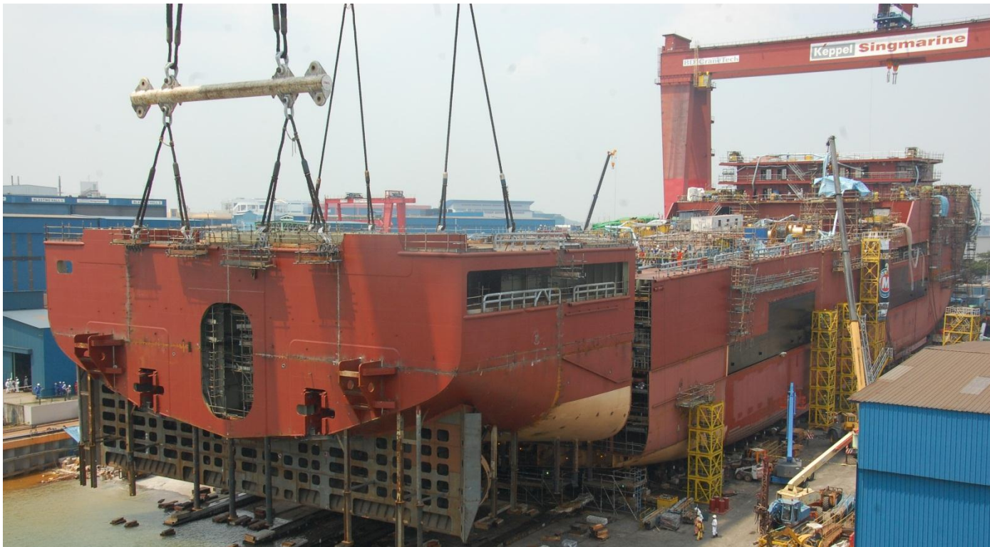
Derrick lay vessel, DLV 2000
