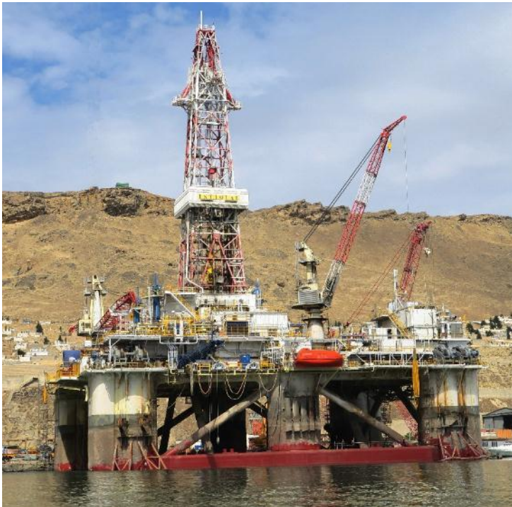
Upgrade of semi drilling rig, Istiglal
