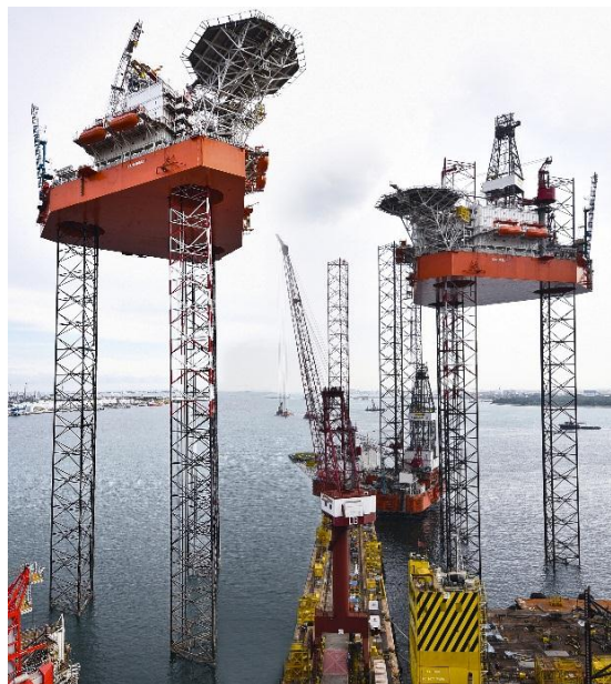
KFELS B Class jackups, CANTARELL I & II
