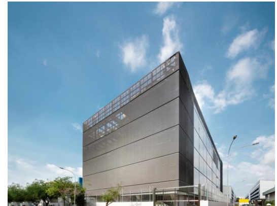
Keppel DC Singapore 4, Singapore
