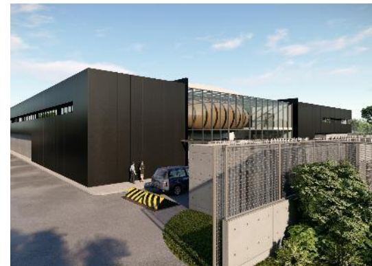
IndoKeppel Data Centre 1, Indonesia
