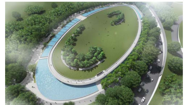
Keppel Marina East Desalination Plant, Singapore
