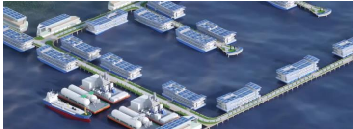
Floating data centre park
