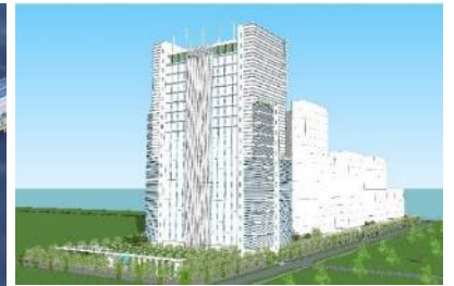
High-rise green data centres
