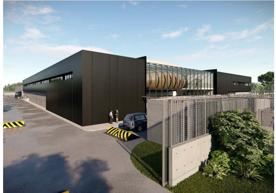
IndoKeppel Data Centre 1 is being developed over three phases
