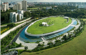
Keppel Marina East Desalination Plant: Singapore's first dual mode desalination plant
