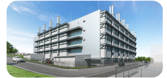
Western Tokyo Data Centre
