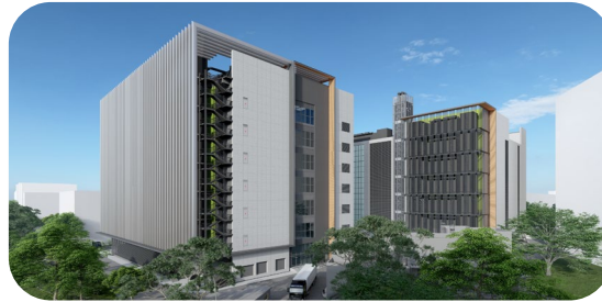
Keppel Data Centre Campus, Singapore
