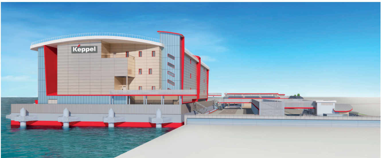
Keppel is pioneering nearshore Floating Data Centres which are mobile, scalable and customisable, to provide a sustainable solution for the growth of the modern digital economy.
