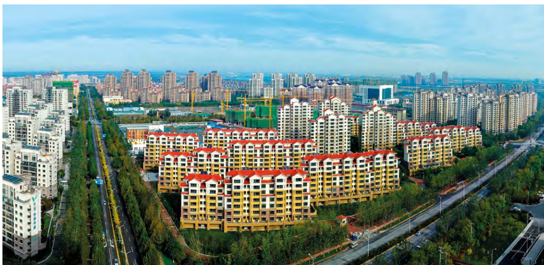
The Sino-Singapore Tianjin Eco-City is on track to realising its vision of becoming a model for sustainable urbanisation.
