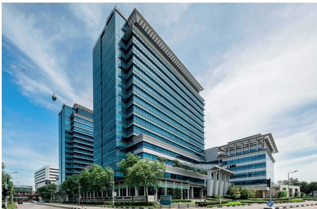
Keppel Bay Tower, where Keppel Corporation is headquartered, is fully powered by renewable energy through on-site and off-site solar power.
