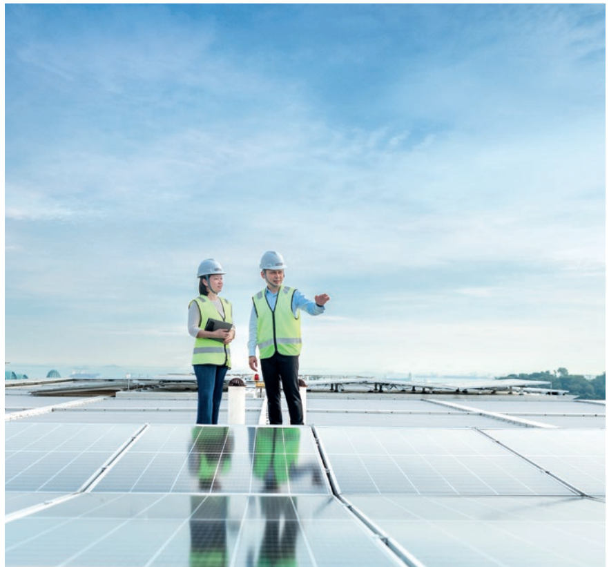
Keppel Bay Tower is the first commercial building in Singapore to be certified as a BCA Green Mark Platinum Zero Energy building. PV panels installed on the roof of the building can generate an energy yield of about 100,000 kWh per annum.
