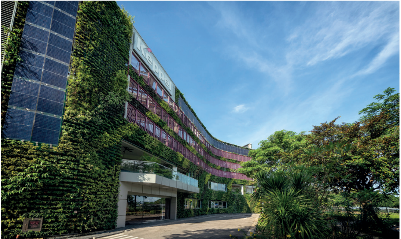
KL@Changi is Singapore's first Green Mark Platinum Positive Energy building under the BCA new Green Mark scheme, and houses our Infrastructure Division's smart operations nerve centre.
